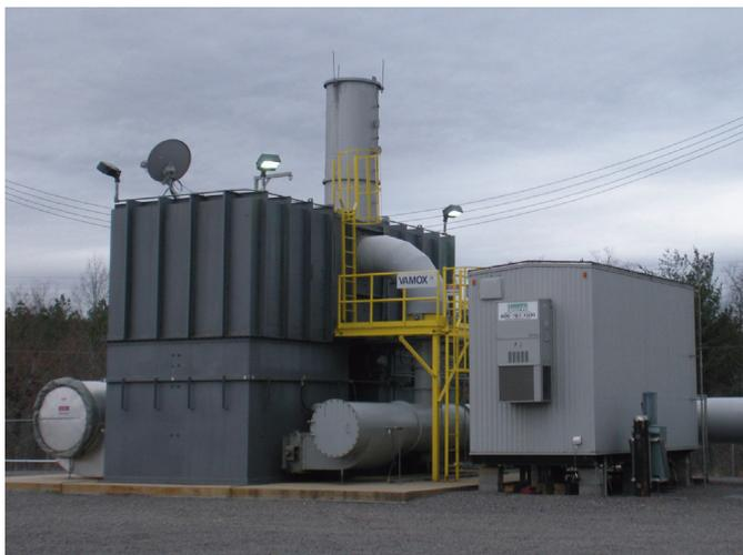
Biothermica's Vamox® system uses regenerative thermal oxidation (RTO) technology to oxidise VAM.
