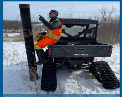
**Biogas Services**Biogas sampling
