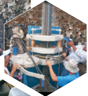
◀ Extension of a vertical well using vertical fusion.
