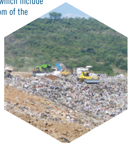
Nejapa landfill site, ▶ El Salvador – waste deposit area
