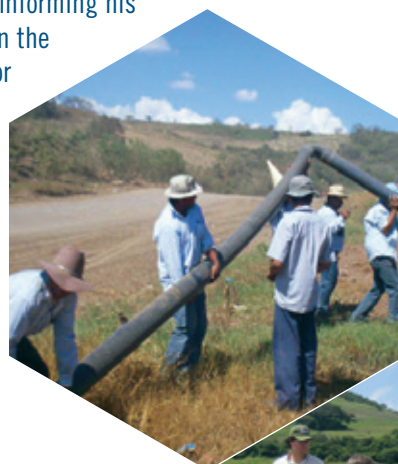
Changing the drainage pipes – from right to left ► - Rigoberto Torres, Mario Torres, Efraín Medrano, Juan Esquivel (sombbrero), Wilfredo Carbajal and Juan Canjura
