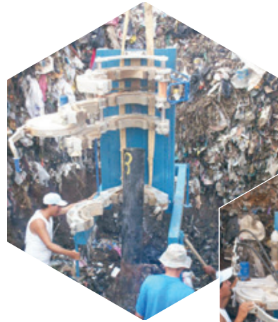
◀ Extension of a vertical well using vertical fusion.
